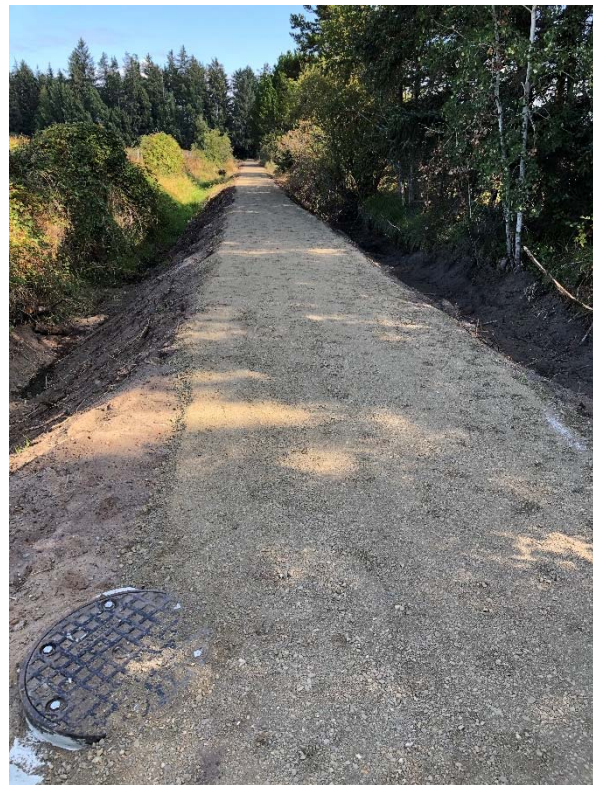
Photo 2- Access path for manholes
