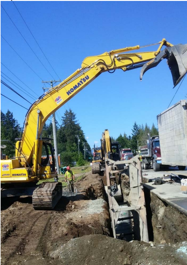
Photo 1- Installation of sanitary sewer along alignment
