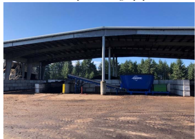
Photo 4- New compost mixing equipment
