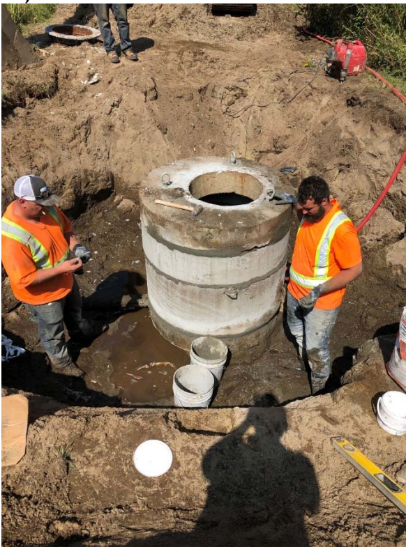
Photo 1- Installation of manhole
