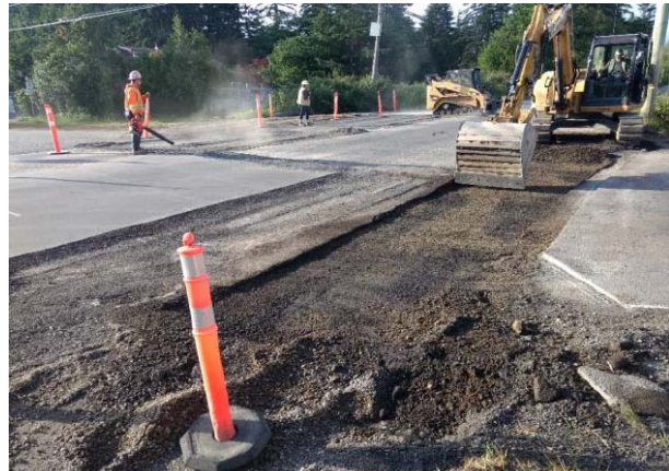
Photo 2- Preparation for paving on Anderton Road
