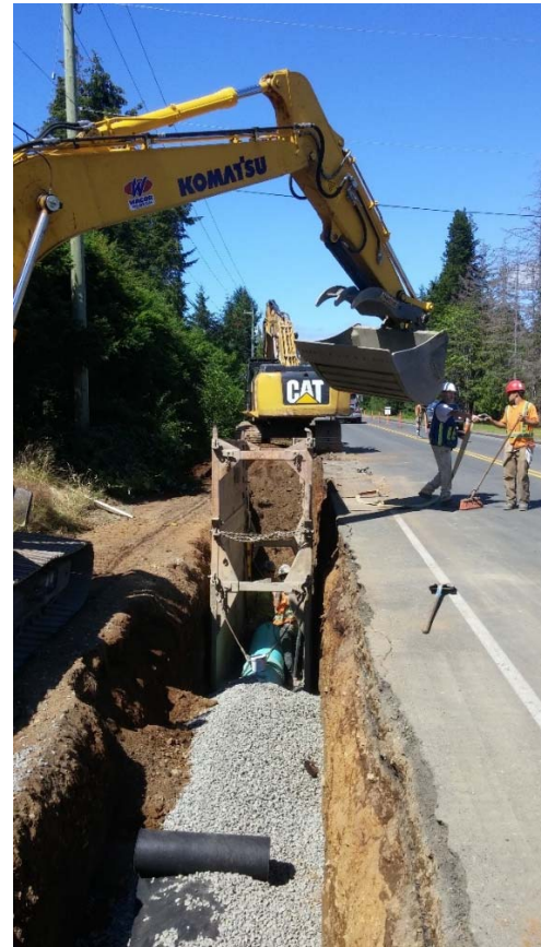
Photo 2- Installation of sanitary sewer along alignment
