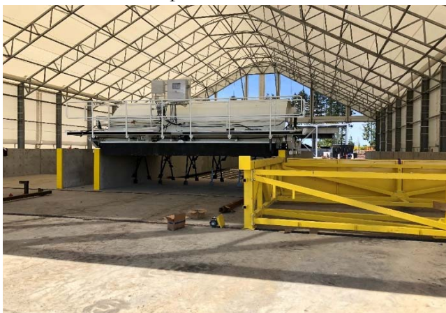
Photo 3- New curing bunkers
